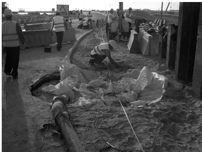
Figure 38.13 A small new sinkhole, already partly backfilled, which developed within a construction site on the coastal sabkha of the Arabian Gulf, after engineering works appeared to have induced dissolution of the gypsum that lies within either the bedrock sequence or the Quaternary cover
