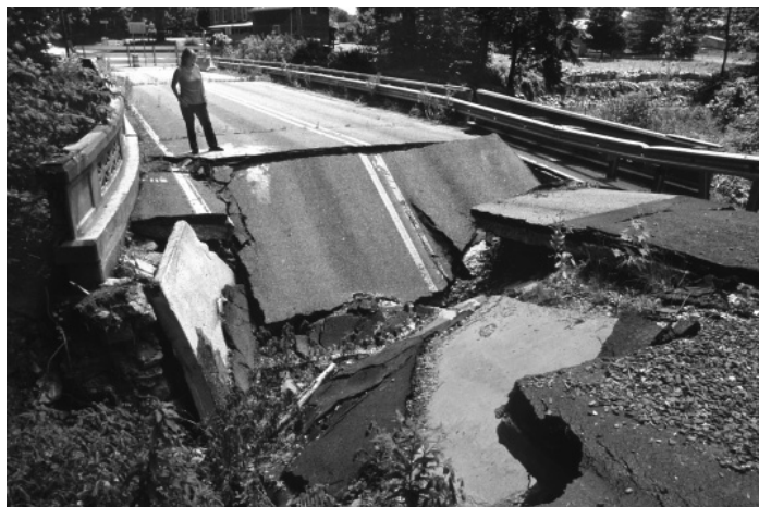
Figure 38.5 Collapse of a road on a bridge approach undermined by a new subsidence sinkhole in alluvial soils in Pennsylvania; this was one of many ground failures that developed within the zone of the decline of the water table around a deep quarry that was kept dry by continuous pumping
