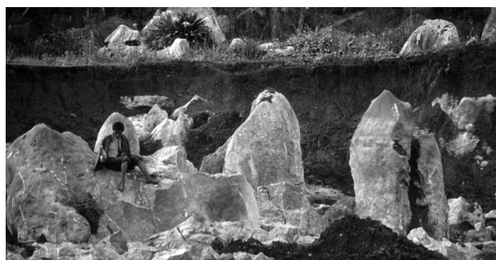
Figure 38.7 Pinnacled rockhead in mature limestone karst (of class kIV), exposed on a construction site in southern China; some pinnacles have already been broken down (with sledge hammers) to create a solid and almost level footing for a new hotel; the grey top of the pinnacle on the right originally projected above the soil level, as do some undisturbed pinnacles in the background
